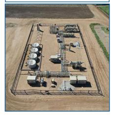
Production facilities are constructed adjacent to the wells to collect and separate the oil, natural gas, and water that are produced. Facility production is 30-45 days of work, completed in stages over about four months.
